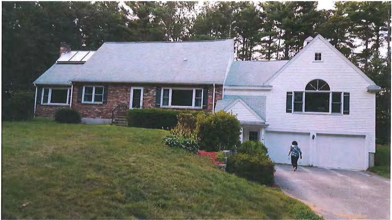
Original structure on left and addition on right.
