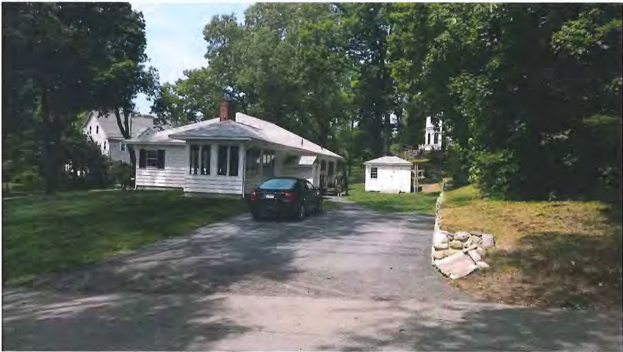
Existing Driveway from Summit Street
