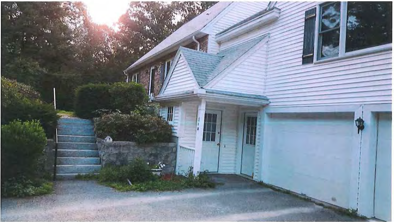
Entry to second dwelling and garage pedestrian entrance.
